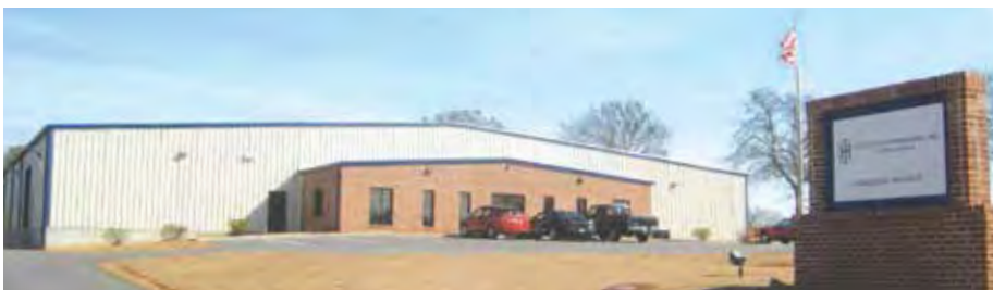
AIRCRAFT COMPONENTS AND GSE MRO FACILITY
